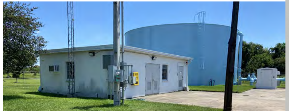
Figure 8-4. Village Drive Water Plant
