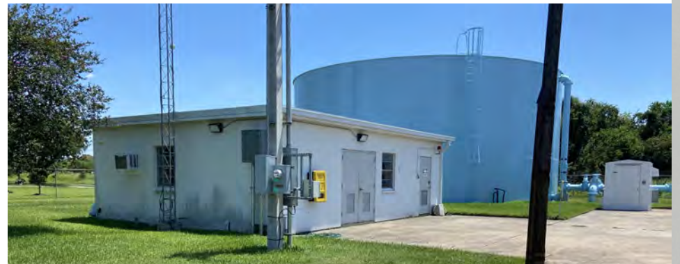
Figure 8-4. Village Drive Water Plant
