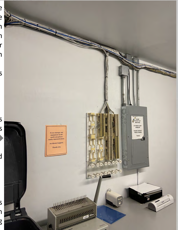
Figure 8-3. Exposed wiring in City Hall
