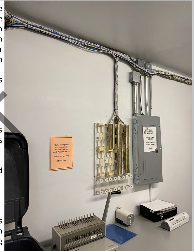
Figure 8-3. Exposed wiring in City Hall
