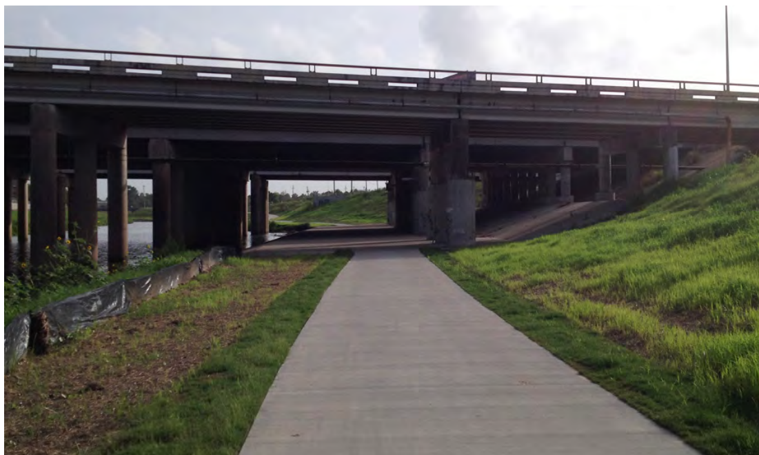
Figure 104. Example of a pedestrian bridge crossing along Brays Bayou in Houston, TX.
