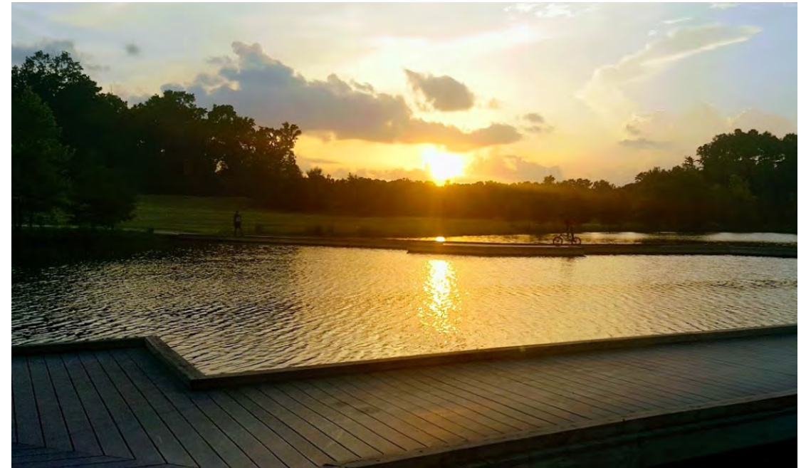
Figure 80.. Example of a boardwalk across a stormwater detention basin at Keith-Wiess Park in Northeast Houston. The project was developed in partnership with Harris County Flood Control District.
