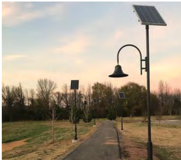
Figure 61. Solar powered lighting can be used along pathways without the need to connect to the electrical grid.
