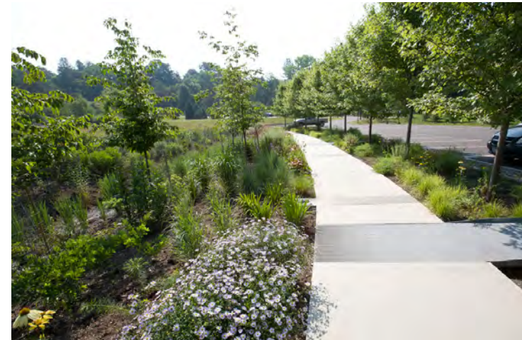
Figure 60. Bio-swales, similar to drainage ditches, utilize selected vegetation to filter and slow down stormwater runoff prior to its drainage into the water shed. These bio-swales can be designed using native vegetation adapted to the area, requiring minimal maintenance.
